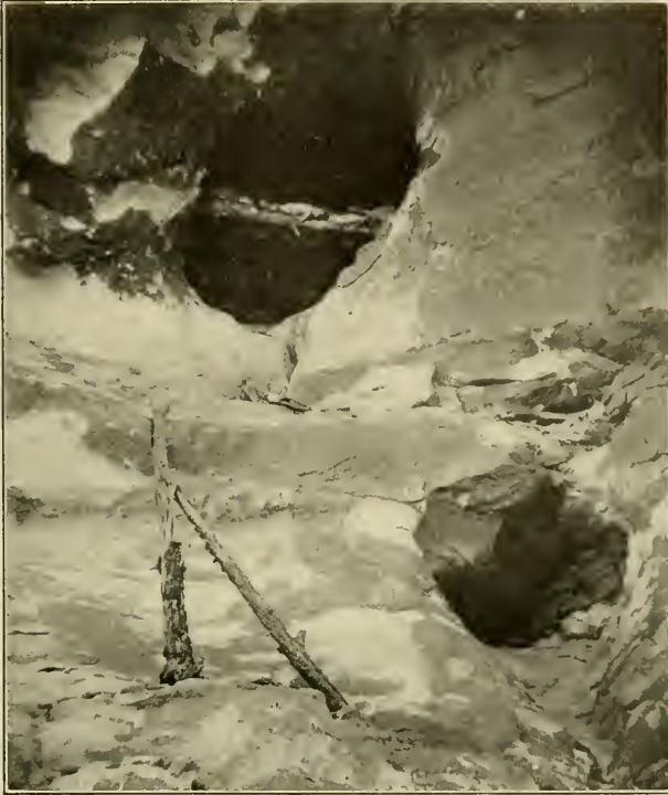
a, SCAFFOLD IN SAND CANYON
