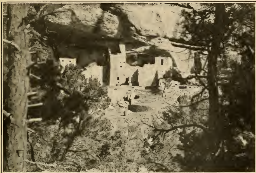
SQUARE TOWER, AFTER REPAIRING
