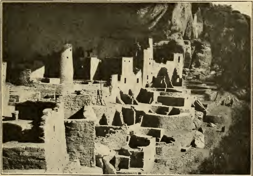
SOUTHERN END, SHOWING REPAIRED TERRACES
