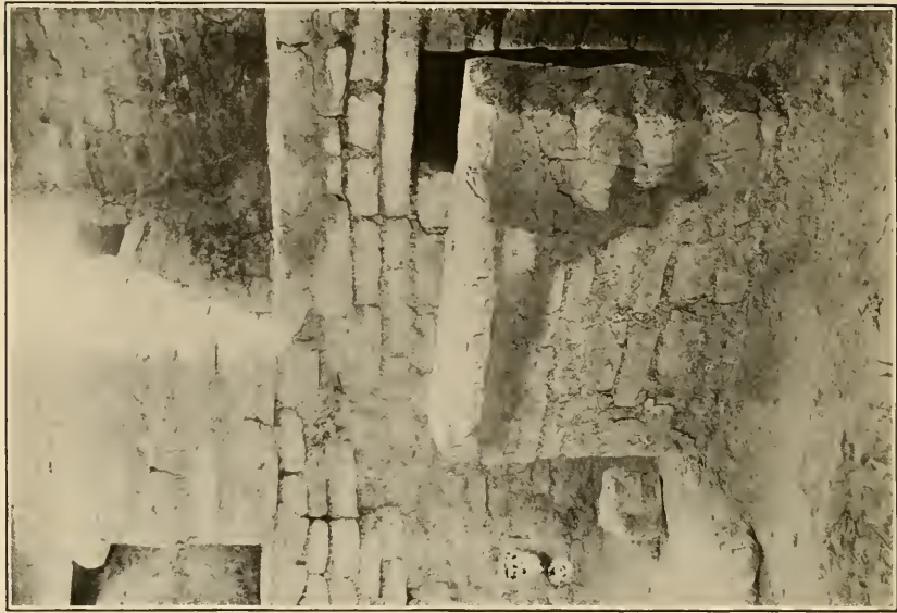
b Deflector and flue of kiva
