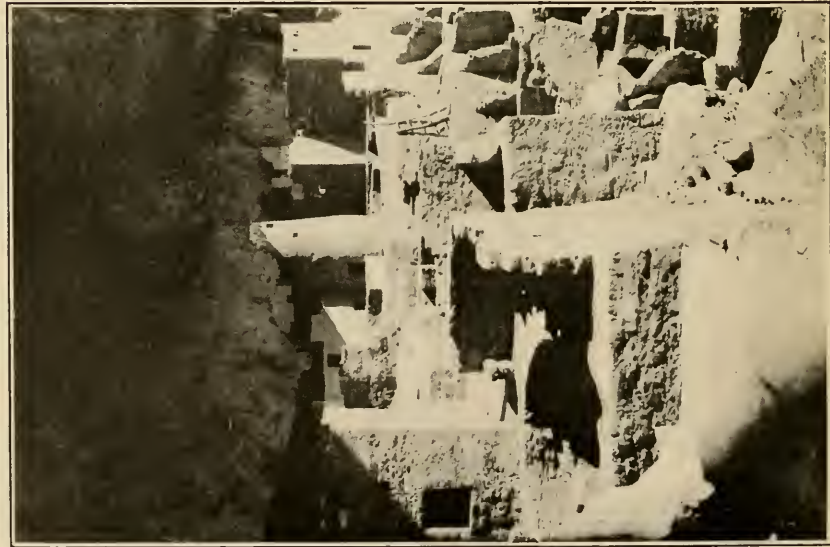
TOWER QUARTER, AFTER REPAIRING
