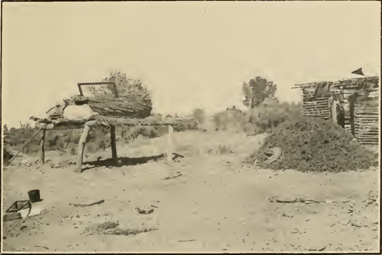
An unfinished house. In the foreground is a pile of screw beans and (on the platform) is a basket therefor
