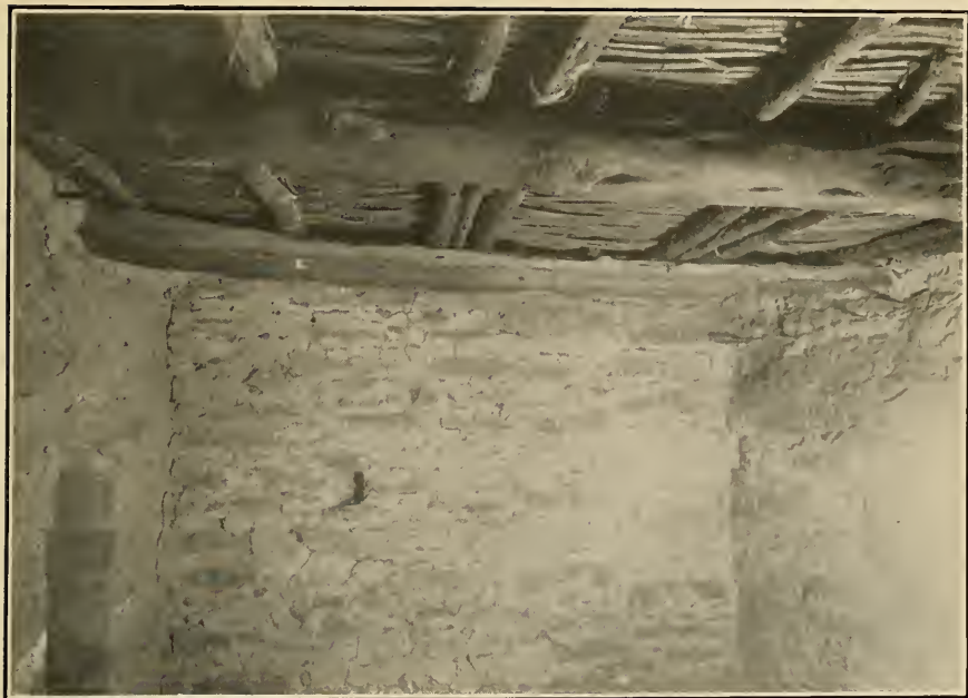
Roof of room 43
