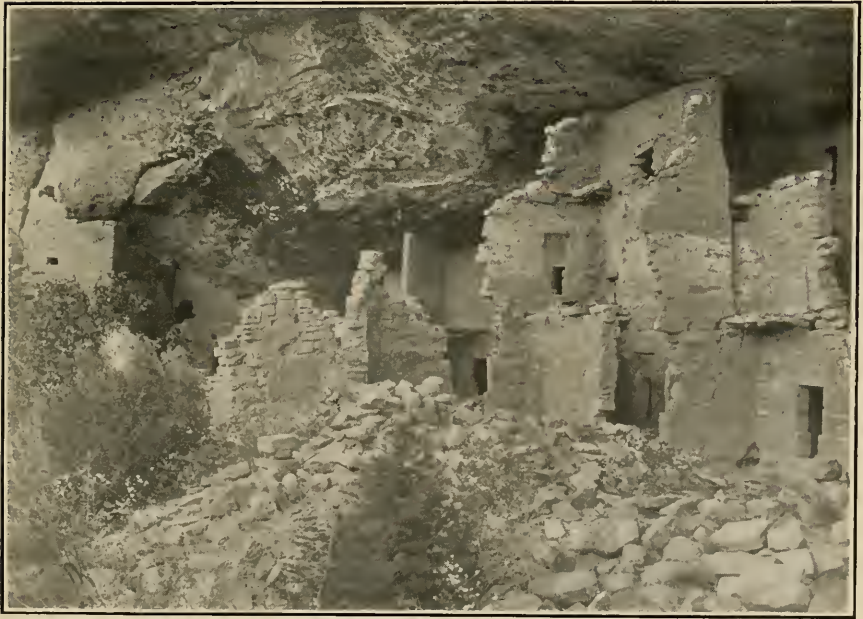
Plaza E. from the south, before repair
