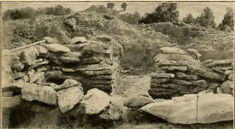
c DOORWAY IN VAULT
