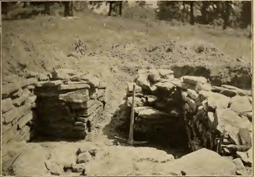
a SOUTH WALL, DOORWAY, AND PASSAGE IN BRENNER MOUND NO. 2
