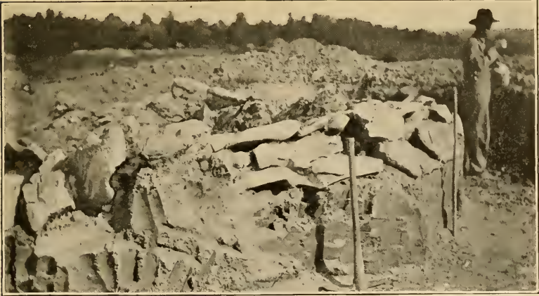
a EXTERIOR OF VAULT
