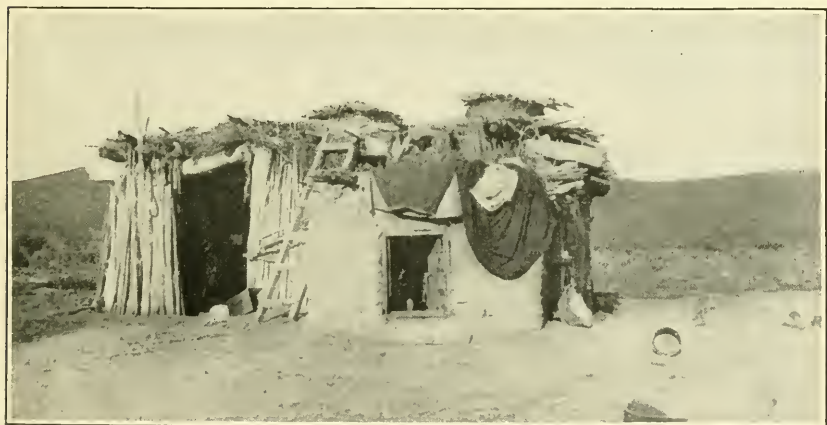
c MADE PARTLY OF ADOBE BRICK
