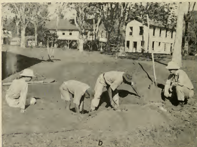
M-1: Mabaruma Headquarters, a habitation site of the Mabaruma Phase. a , General view showing the main street and government buildings over the central part of the site. b , Excavation of Cut I in the front yard of the guest house. Osgood's excavations in 1944 were to the right of the two-story building.
