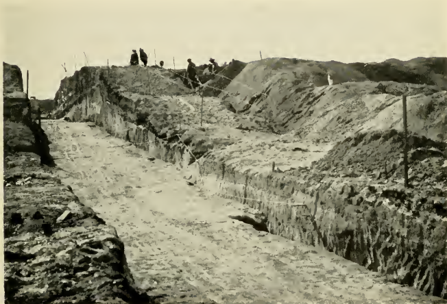
a , North wall of trench 1, site 1, from lake bed.
