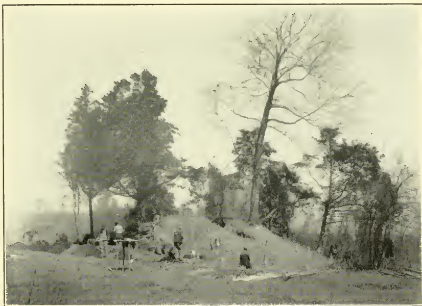
b , Excavation starting, Site La° 37.
