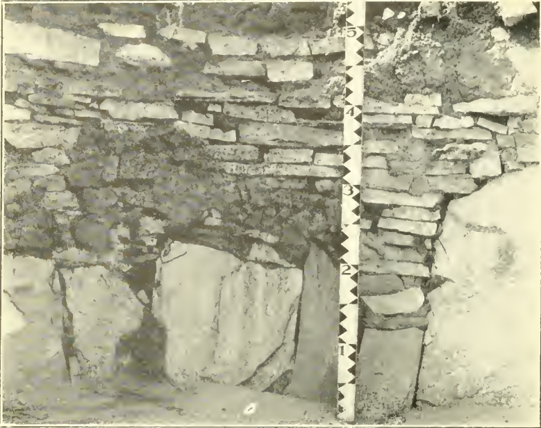
a. Masonry wall resting on slab foundation.
