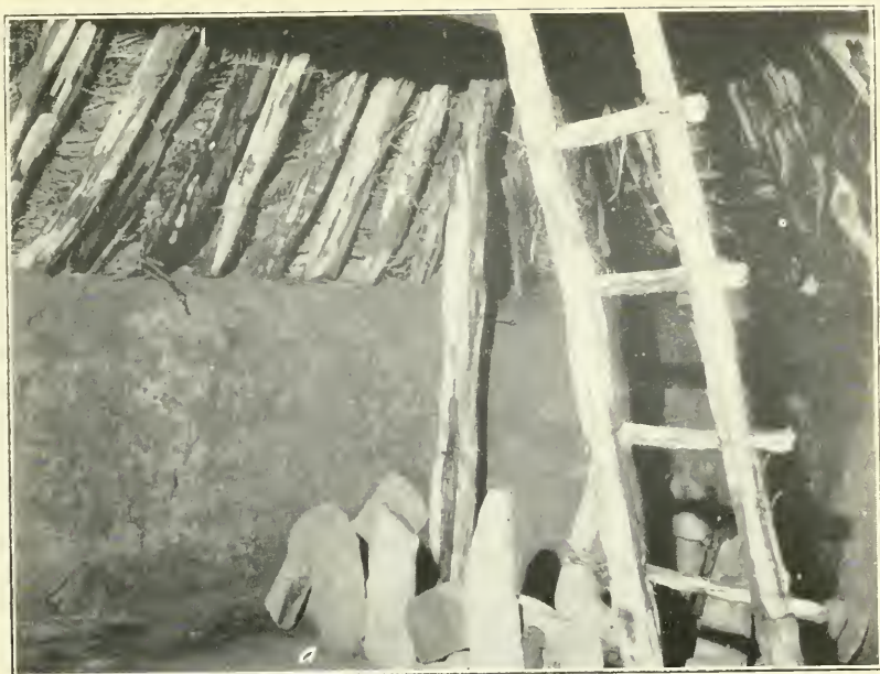
a. Interior view of portion of restored structure.
