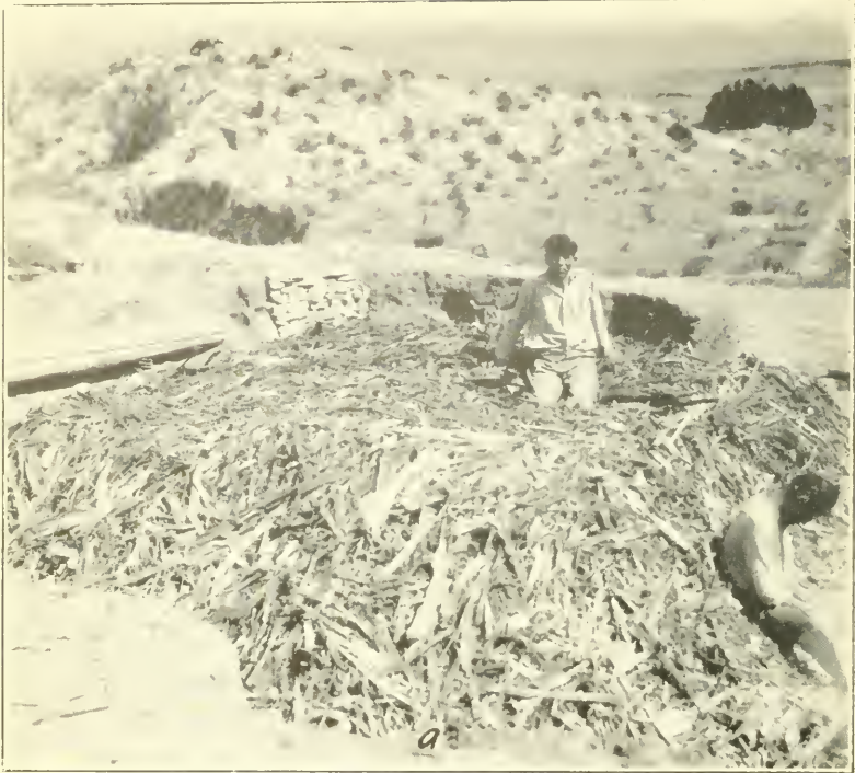
a. Brush-and-bark covering over framework, restoration of structure 1.
