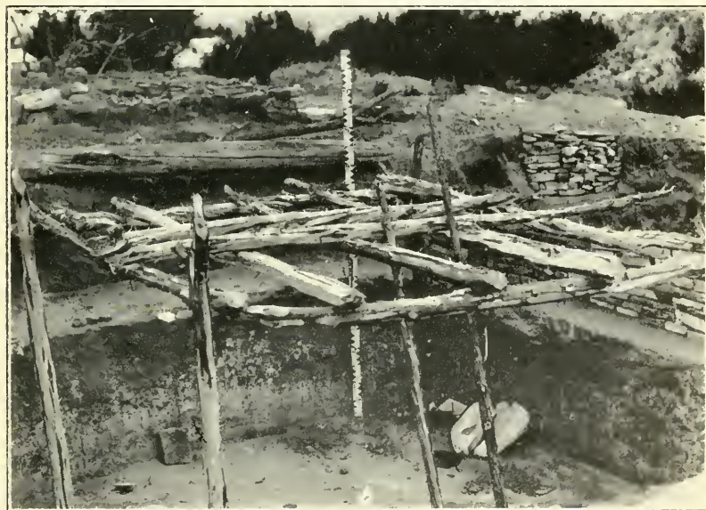
b. Main framework for restoration of structure 1.
