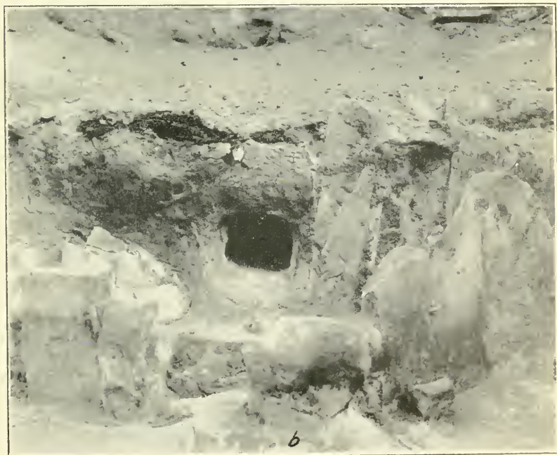
b. Compartment wall and ventilator of structure 15.
