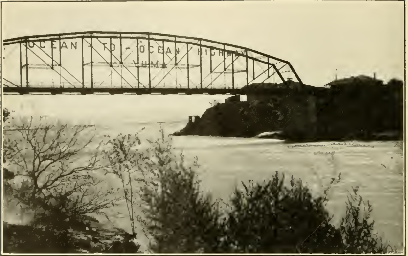
a. BRIDGE ACROSS COLORADO RIVER AT YUMA
