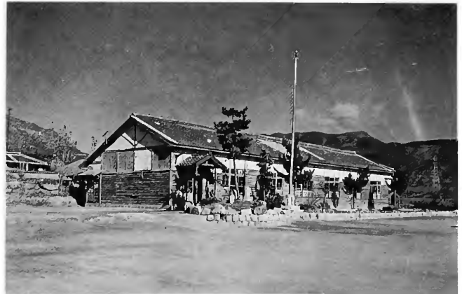
FIGURE 15.—The Sam Sung primary school in Three Ministers village. Suh Sul-Bong, an elder in Three Ministers village, working with a U.S. Army engineer (Lt. Col. ? Ellis), built this primary school along with others throughout the Kimhae area. U.S. Army advisors were stationed in Kimhae with the Korean Army Engineer School, 1945–1948. Black and white photograph, 1953.
