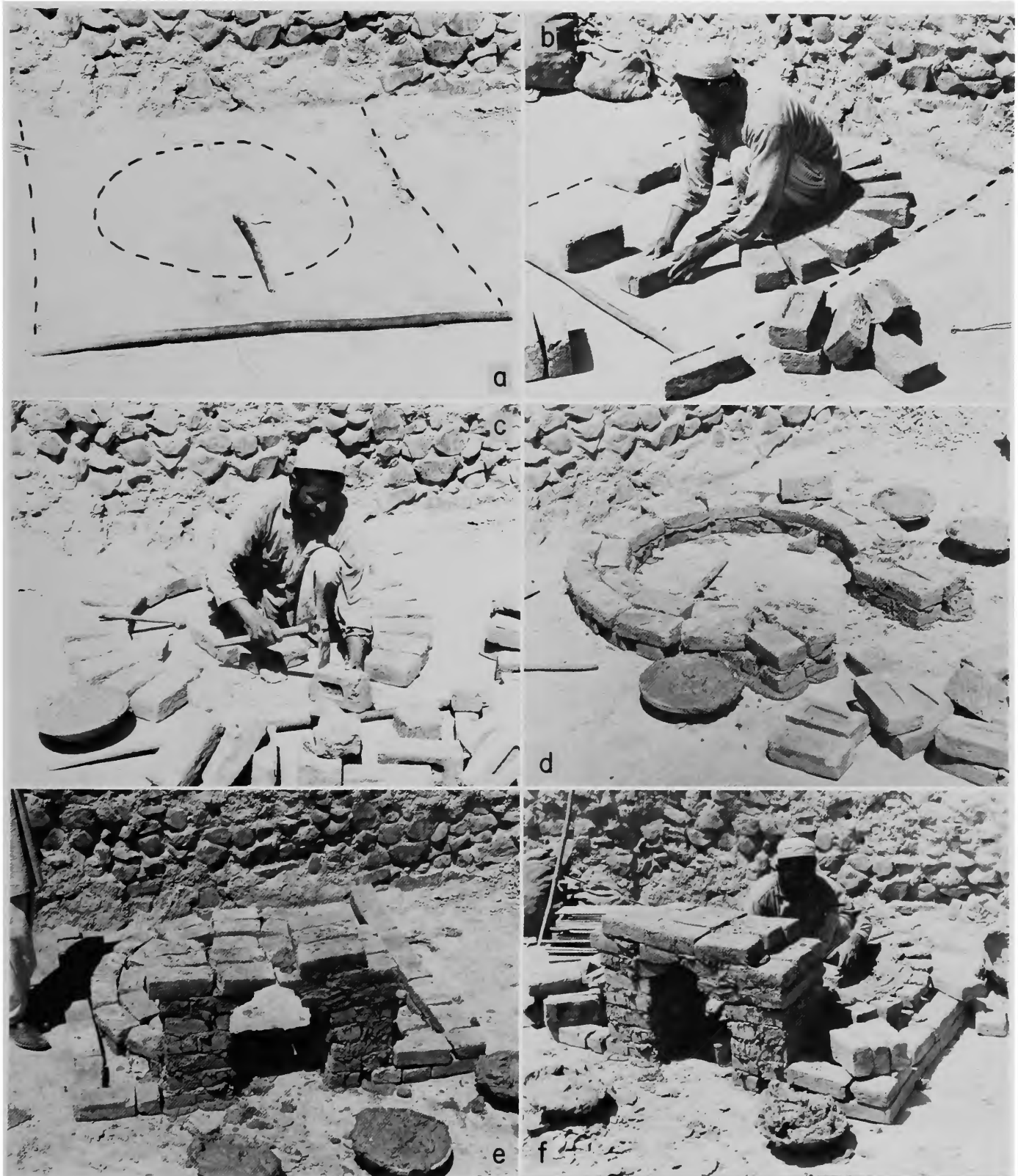
PLATE 62.—Potter Roshan Din demonstrating kiln construction, Zakhel Bala, NWFP: a , stick in foreground used to measure dimensions of kiln plan (broken lines); b , setting out position of stokehole; c , method of cutting bricks with an adze-like tool; d , first two courses of the firebox and stockhole completed; e , stockhole, closed by corbelling, completed (first courses of outer insulating wall laid); f , commencing construction of firebox. (See Plate 63.)
