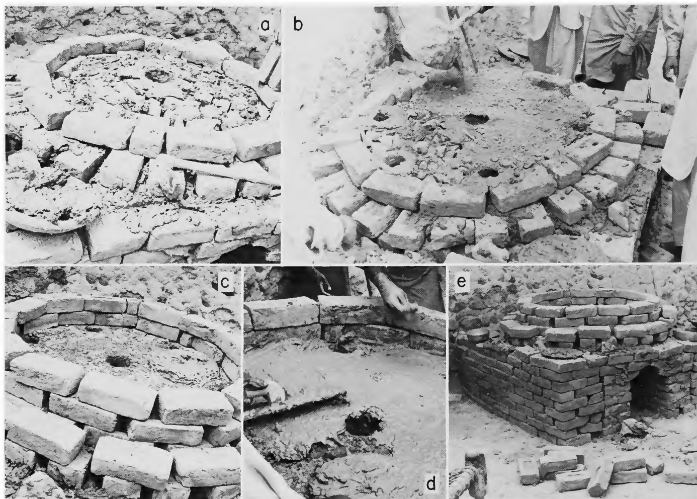
PLATE 65.—Potter Roshan Din demonstrating kiln construction, Zakhel Bala, NWFP (continued): a , chamber floor (dome over firebox) brickwork completed; b , flamethroats (openings) built up with plastic clay, then dry clay shoveled in to level floor; c , water has been sprinkled on dry clay; d , wet clay is trowelled over floor to smooth and level it; e , kiln completed to chamber floor level (the circular brickwork will be continued upward to form the chamber; the square outer wall will be continued upward to form the outer insulating wall; formwork (steel drums, wood, dry clay) is removed from under floor through the stokehole at front).
