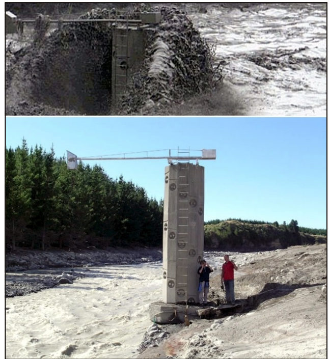
Figure 13. Comparative photos of the 6.2-m high OnTrack (New Zealand Railway Corporation) lahar warning tower, located in the Whangahu river 28 km downstream from Crater Lake. The tower was installed following the 1953 Tangiwai disaster to provide 15-min warning for the railway bridge 11 km downstream. The arm on the tower supports a radar stage gauge to measure flow depth. Images were captured by a Horizon Regional Council web cam. (top) Tower in the path of the lahar flow at 1255 on 18 March 2007. (bottom) Examining lahar deposits on 21 March 2007, with researchers providing scale of the tower and its inscribed scale marks. Courtesy of GNS Science and Vern Manville.
