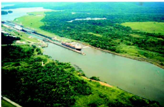
Figure 3. Gatun Locks aerial view looking southwest from the Caribbean entrance to the Panama Canal. This is the largest set of locks (approximately 2 km) with 3 levels and 6 functional chambers designed to raise or lower vessels by 26 m above sea level (photo by Marco Guerra).
