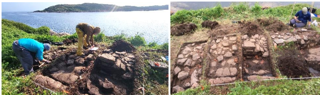
Kody and Alyssa working on the foundation units at the southern end of BE-4. View SW. (photo: Sofia Vakhunitsky); Units 15-18 South with the stone foundation at 2 West, view W.
