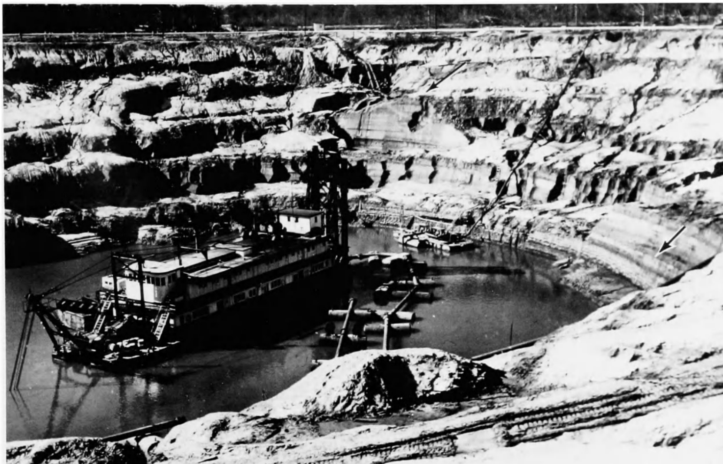
FIGURE 23.—Test pit at Texasgulf Inc. Lee Creek Mine. Water level is at middle of Pungo River Formation with 96 feet (29 meters) of section exposed. Arrow near right margin indicates contact between Pungo River and Yorktown formations in face; close-up of face is shown on Figure 24. Two clean faces in center above lowest bench are in lower and middle parts of the Yorktown Formation. Arrow in upper center indicates boulder beds or unit 7 of Gibson (1967), now considered in lower part of Croatan Formation.
