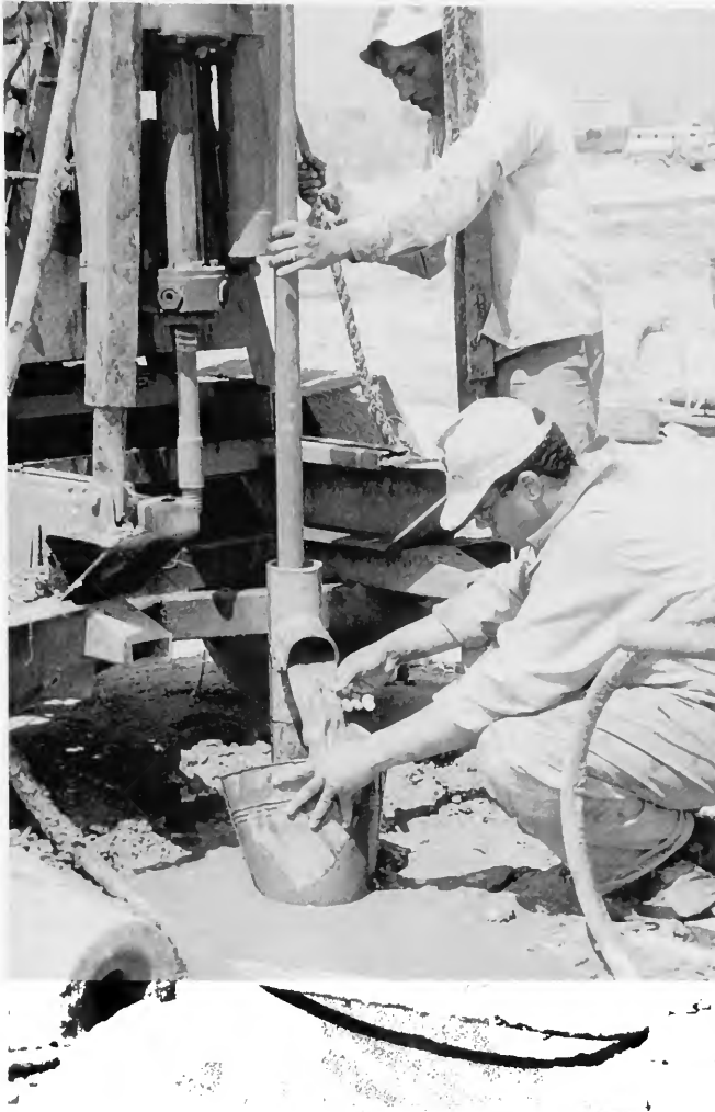
FIGURE 5.—Recovery of sediment from washings of circulated water in a thick sand sequence. Photograph taken at site S77 in September 1990.
