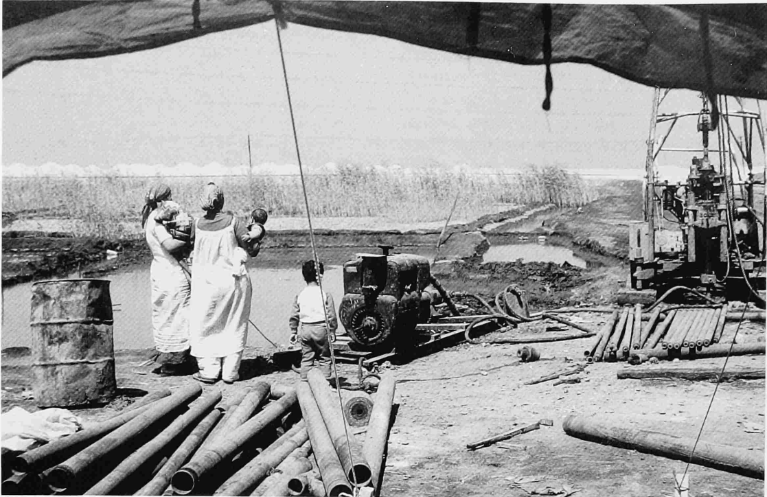
FIGURE 3.—Large-diameter pipes in foreground are used for casing, particularly when drilling in thick sections of sand and/or soft mud. Note 10-foot (3.05 m) lengths of drill pipe assembled near the drilling equipment. Photograph taken at site S11 in September 1985.
