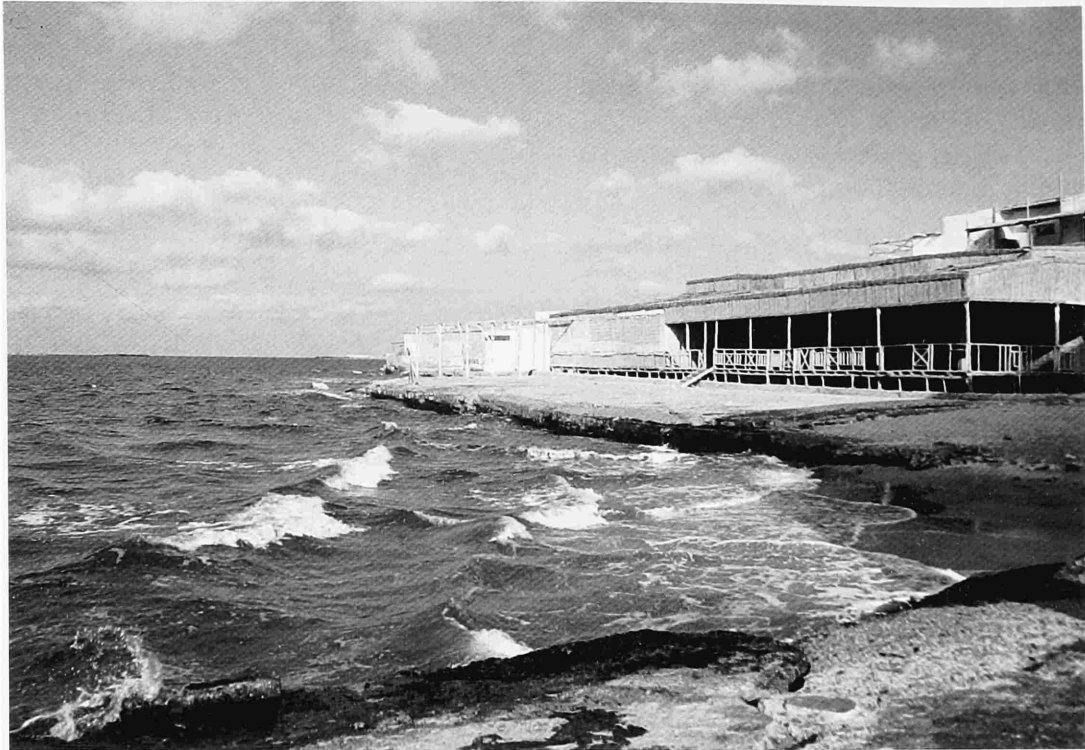
FIGURE 10.—Section of the town of Ras El-Barr at the Damietta promontory (north of Damietta, D on Figure 1), recently abandoned and undergoing destruction by intense coastal current erosion. Relatively rapid incursion of the sea in this region is due to concurrent subsidence of land and rise in sea level as indicated by analyses of radiocarbon-dated drill cores. Photograph taken in October 1992. (Courtesy of G. Drapeau.)
