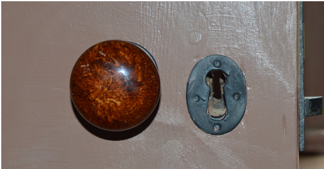
FIGURE 18. Front of the door of the small bedroom, showing the original brass escutcheon plate around the keyhole, which has been incompletely recut to match the later Russell and Erwin lock, leaving wood at the bottom of the keyhole.
