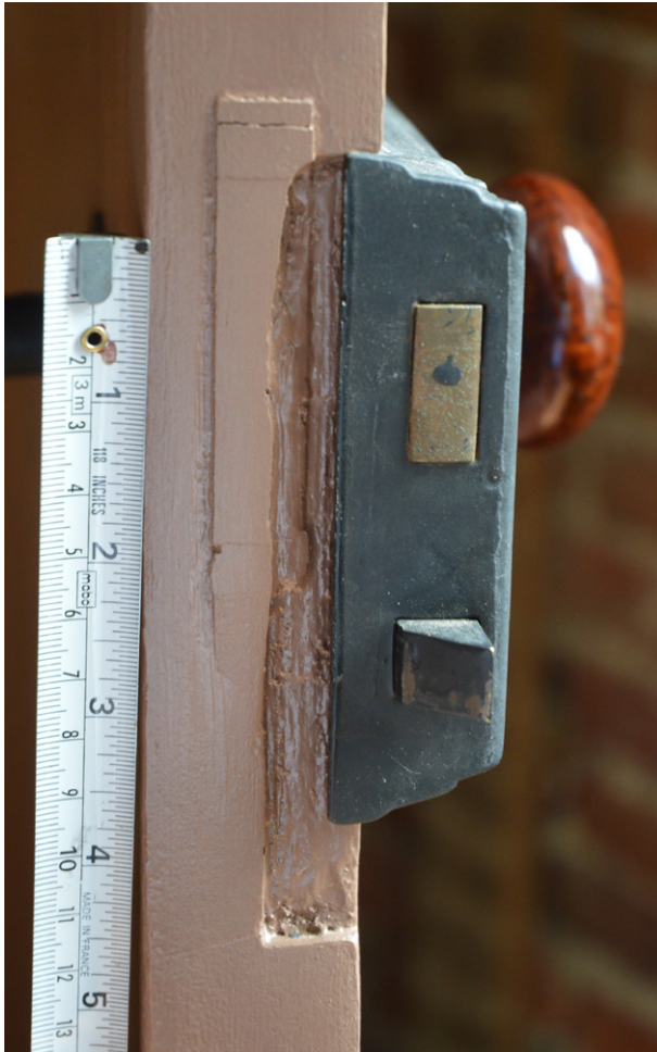
FIGURES 19-20 (left to right). (19) Side view of the Russell & Erwin lock on the small bedroom, showing earlier cuts for the Carpenter lock at the bottom and side. Although the Russell & Erwin lock is smaller, its configuration required that it be placed slightly higher, as can be seen by its position relative to the tongue of the rail when compared to that of the lock in the following figure. (20) Side view of the same-sized Carpenter lock on the master bedroom door as the corroded lock.
