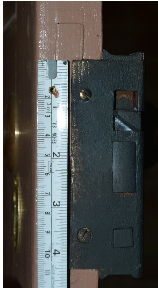
FIGURES 19-20 (left to right). (19) Side view of the Russell & Erwin lock on the small bedroom, showing earlier cuts for the Carpenter lock at the bottom and side. Although the Russell & Erwin lock is smaller, its configuration required that it be placed slightly higher, as can be seen by its position relative to the tongue of the rail when compared to that of the lock in the following figure. (20) Side view of the same-sized Carpenter lock on the master bedroom door as the corroded lock.
