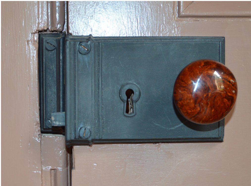
FIGURE 16. Small bedroom Russell & Erwin lock currently on the door of the small bedroom (25 June 2021). Note the gap in the molding below the keeper at left, which reflects the larger size of the original Carpenter lock keeper.
