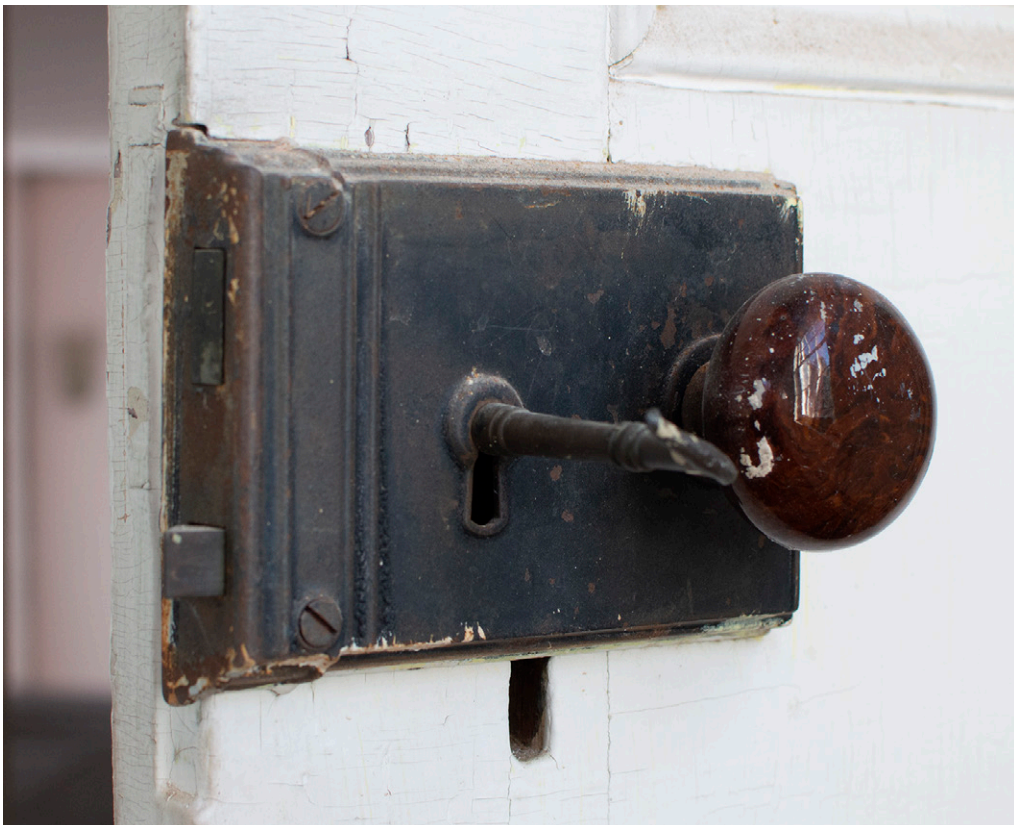
FIGURE 17. Small bedroom lock image 3.182 from the 2017 Historic Structure Report, showing part of the original keyhole for the Carpenter lock below it.
