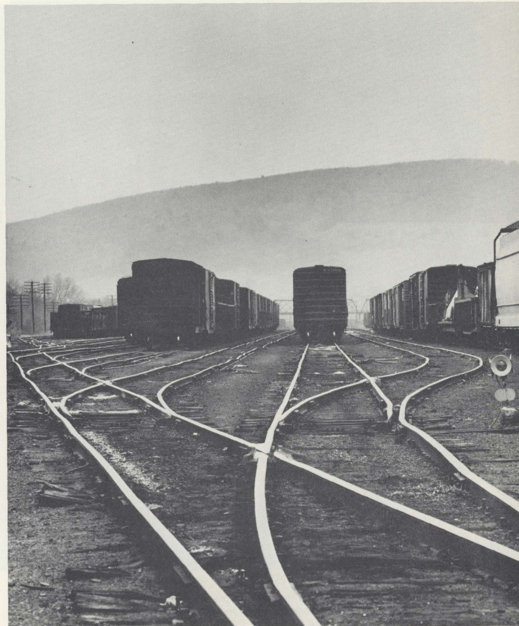
Ladder track in a freight classification yard
