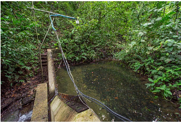
FIGURE 3 Photograph of Lutz Creek V-notch weir, Barro Colorado Island
