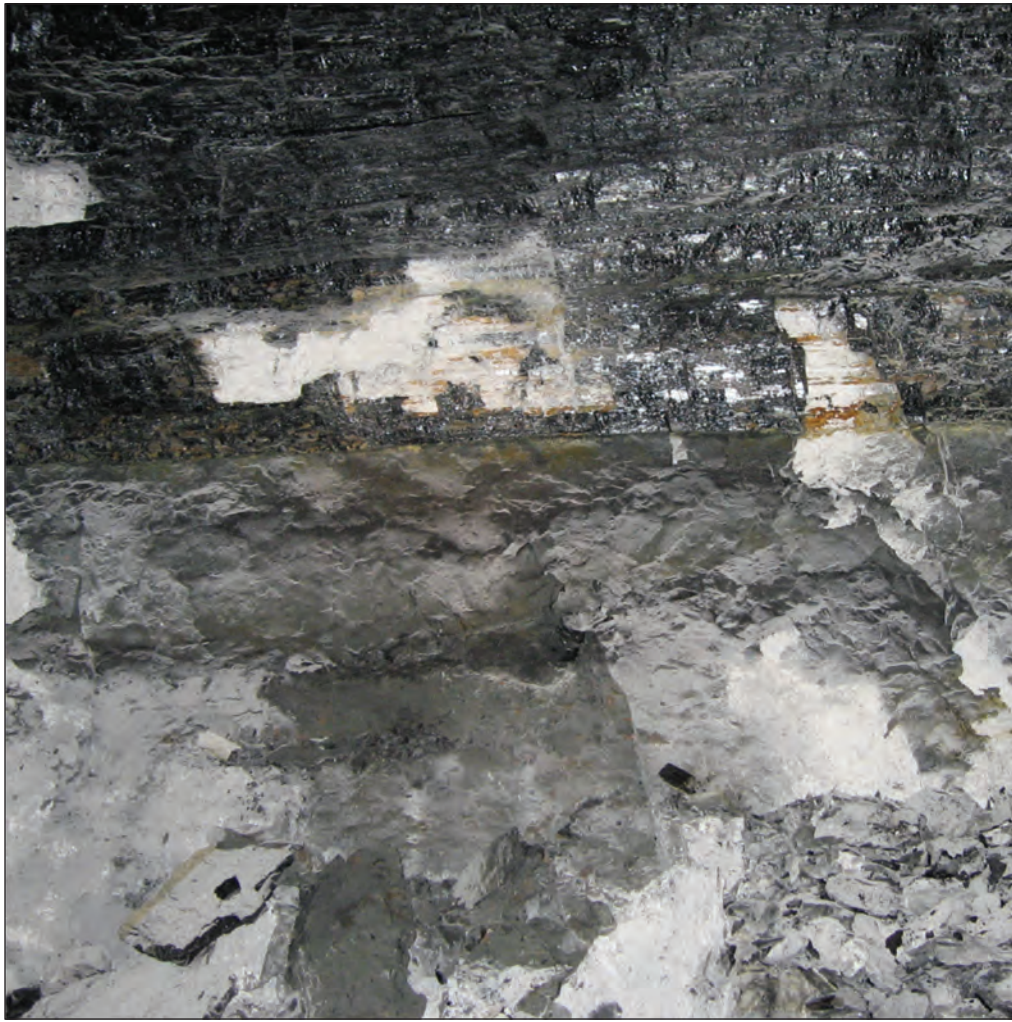
Figure 9 Photograph showing underclay of the Springfield Coal at American Coal's Galatia Mine, Saline County, Illinois. Field of view approximately 5 ft (1.5 m) square.
