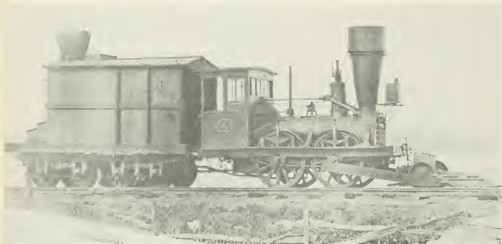
Figure 33. — As this early photo shows, the John Bull toward the end of its active career had a cab and large smokestack, and an 8-wheeled tender was used.
