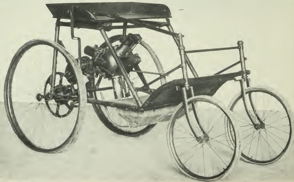
Figure 38.—This 1894 Balzer automobile had a 3-cylinder rotary engine.
