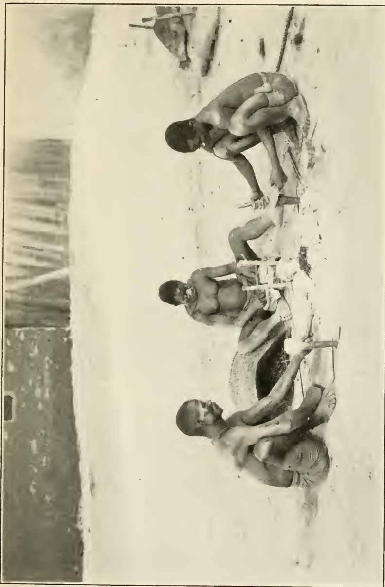
ANGOLA NATIVE BLACKSMITH AT WORK, USING A TWO-PHASE BELLOW
