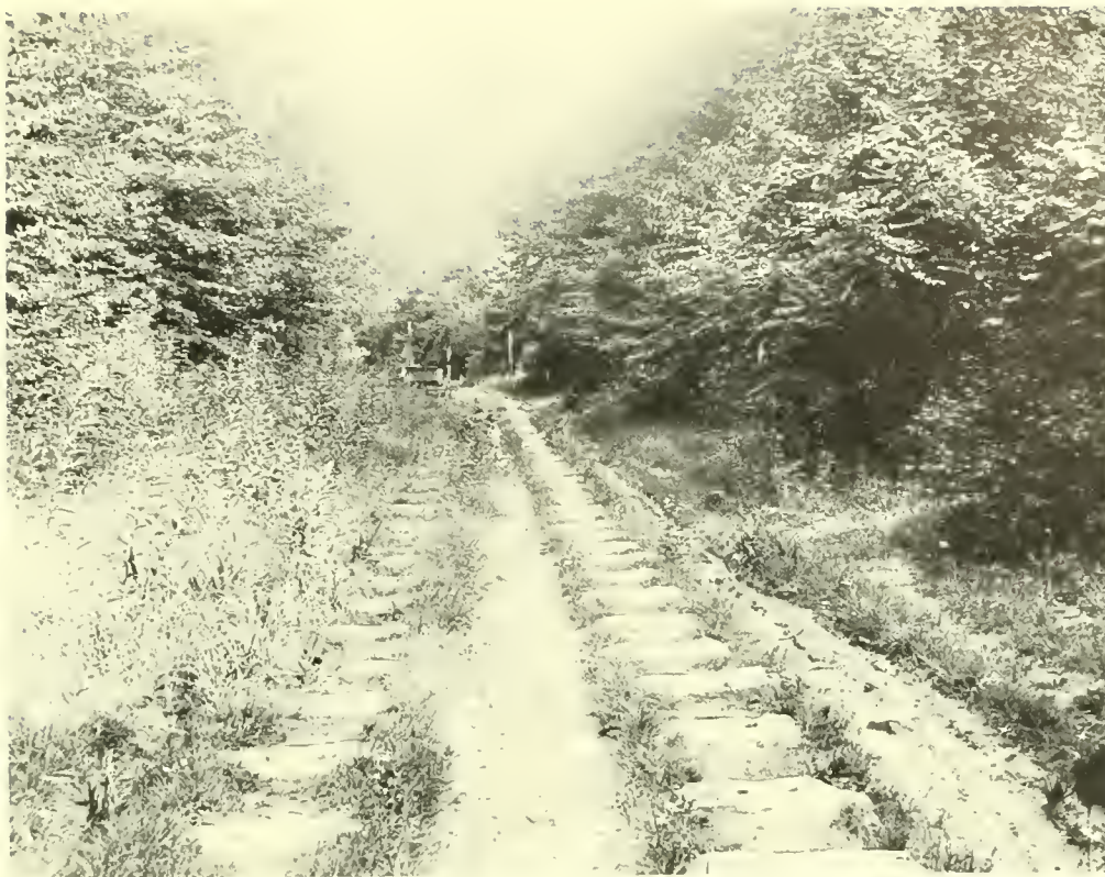
FIGURE 63.—Roadbed of abandoned Portage Railroad. Note the closely spaced granite blocks. From an original photograph in division of transportation, Smithsonian Institution.
