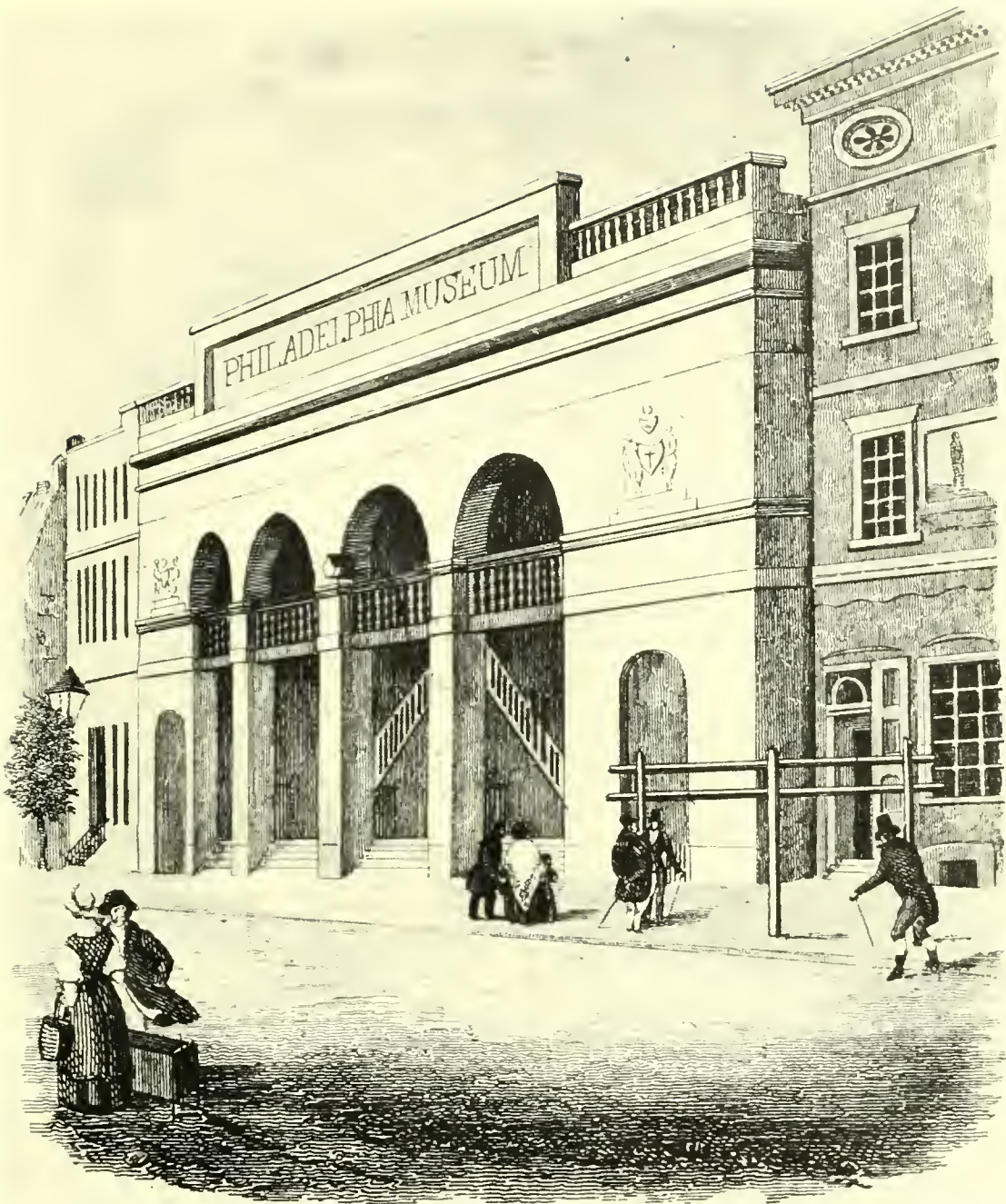
FIGURE 33.—Arcade Building, Philadelphia, located on Chestnut Street near Sixth. Designed by John Haviland, this building was completed in 1827. There were three floors, the first two having some 80 shops open to arcades; the museum was located on the third floor. From Traugott Bromme, Genälde von Nord-Amerika , 2 vols. (Stuttgart, 1842).
