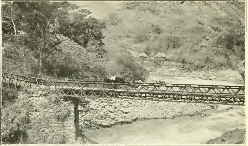
CHAULLAY BRIDGE OVER THE URUBAMBA RIVER.
