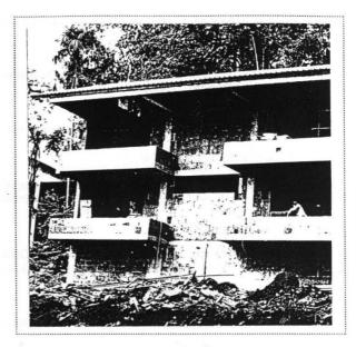
One of the new four-apartment dormitory buildings on BCI. All the roofs have been installed, and the contractor is plastering the walls, installing floor tiles and door frames.
