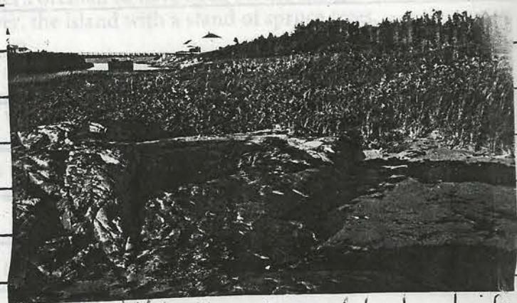
Kegashka Is. toward harbor bridge
