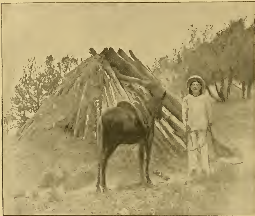
FIG. 238—A timber-built shelter
