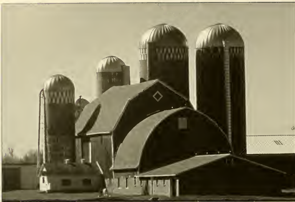
The gambrel-roofed barn, gothic-roofed barn, and pole barn (from left) on this farm demonstrate both the change in style and continued usefulness of older structures. As farms grow and change, barns are added, not replaced. Photo © Bob Rashid
