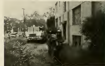
4 Taking the hose line into the building
