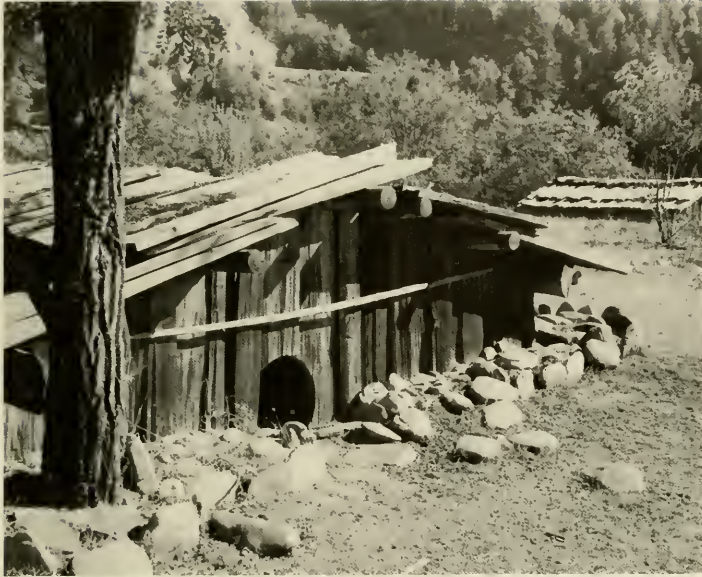
The Hupa of Northwestern California utilize earth as an insulating material by building semi-subterranean plank houses. Photo by Peter Nabokov
