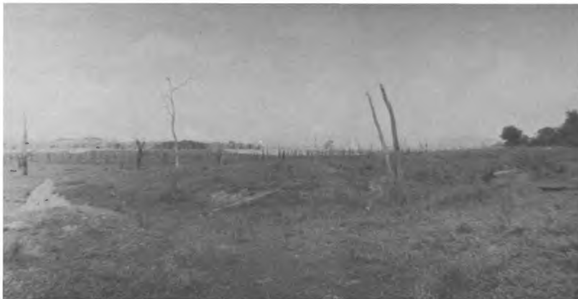
FIGURE 13.—Upper bank of Senanyake Samudra at Kossapola. Note the presence of a few dead trees on the upper bank. At the time this photograph was taken (1968) this section of bank had been dry for several years and termites had invaded from the forest.
