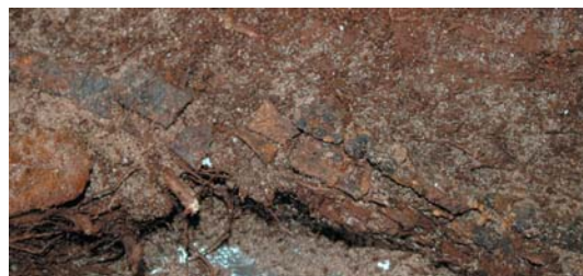
Fig.8 Detail of iron pieces exposed in the central area near the base of the wall [4 July 2006]
