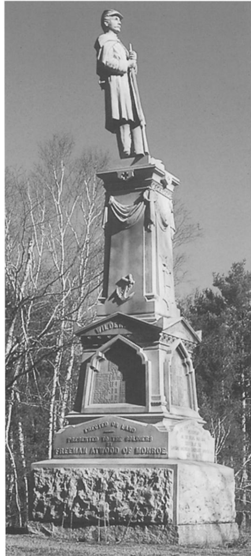
Fig. 5. The Monumental Bronze Company's Civil War Monument (1887), showing the soldier's pronounced backward lean, white bronze, Monroe, Maine. Photograph by Ronald S. Harvey
