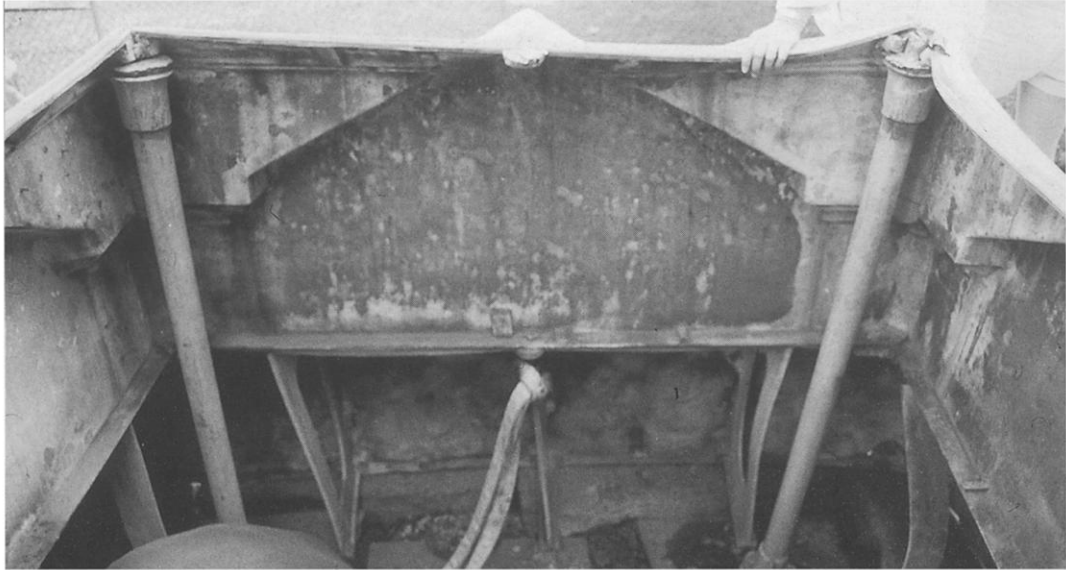
Fig. 8. Interior of lower sections of the Monumental Bronze Company's Settlers' Monument (1889) during disassembly, showing the original corner posts and buckled vertical stiffeners, white bronze, Newark, N.J. Photograph by Carol A. Grissom
