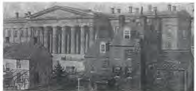
Figure 4. South Aquia Creek sandstone wing of the Patent Office Building by John Plumbe, around 1846 (courtesy, Library of Congress).
