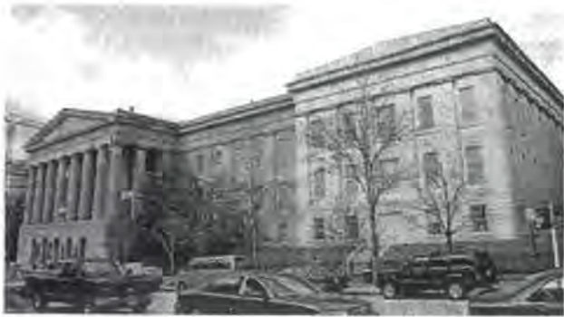
Figure 1. The former US Patent Office Building, Washington, DC, from the southeast (March 2000). The original Aquia Creek sandstone wing is on the left, and a later Texas marble wing, on the right.
