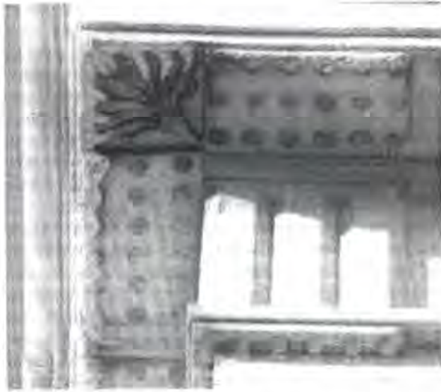
Figure 7. Detail of Texas (Maryland) marble cornice on the later west wing.
