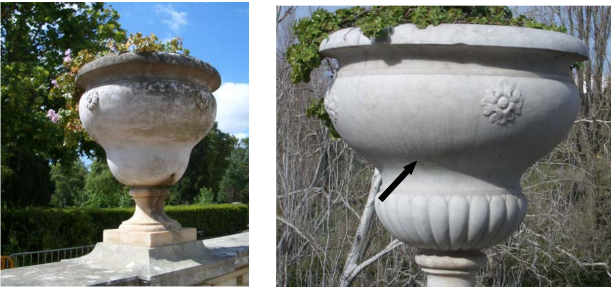
Figure 5: (a): A marble vase on the same balustrade of the putti from Fig.3 that did not receive a water repellent treatment. Note the even biological colonization that is mainly favoured by the orientation of the object. (b): A marble vase located on the balustrade of a sunny terrace, cleaned and treated with the aqueous water repellent emulsion in 1999, shows the resulting tell-tale streaking nine years later (Photo 2008).
