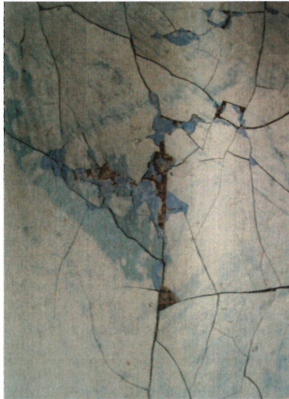
Figure 2 Detail of a painting by Henry Cliffe (1959). The paint shown in this detail is lead white containing zinc. Note the severe cracking and interlayer cleavage. This is mechanical damage due to rolling and not to moisture or temperature effects. (Photo: Steve Gayler. Courtesy of the owner, Richard Saltoun.)
