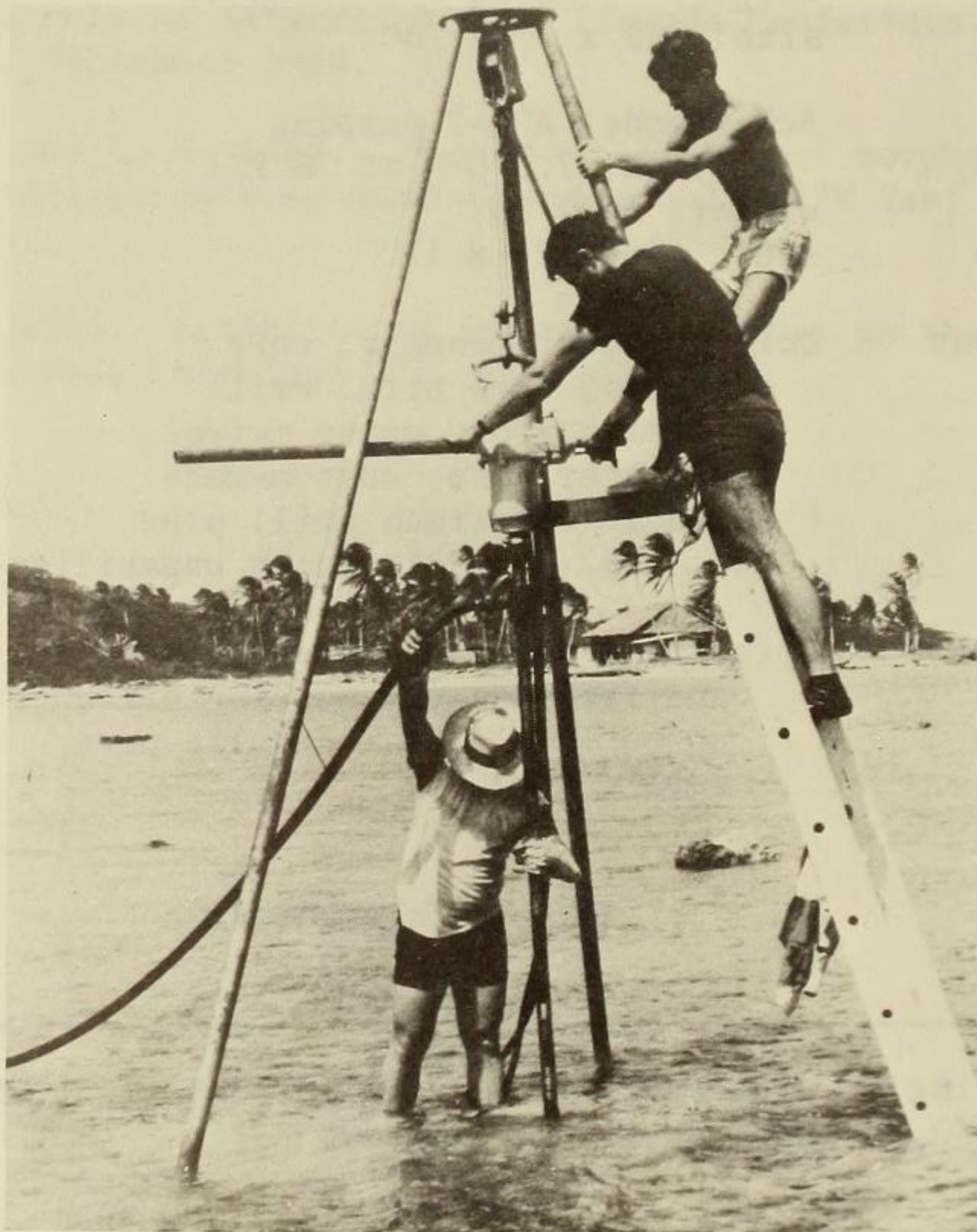
Figure 2. Tripod-winch assembly. Galeta Point, Caribbean coast of Panama. Note pipe braced against leg of tripod and trigger control at operator's right hand.
