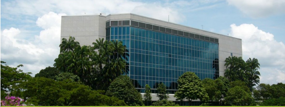
The Administration Building of the Nanyang Technological University in Singapore. (View from the North Spine)
