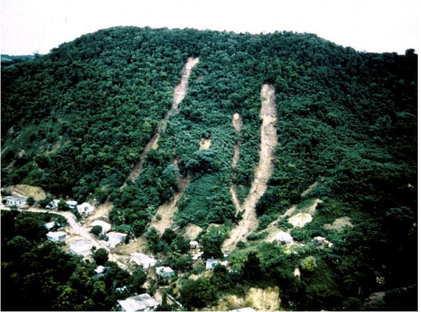
Figure 5. Vulnerability to debris flow hazard of homes and other structures at the base of steep hillslopes such as this one in Penuelas, southern Puerto Rico. Photo source: R. Jibson, USGS, 1985.
