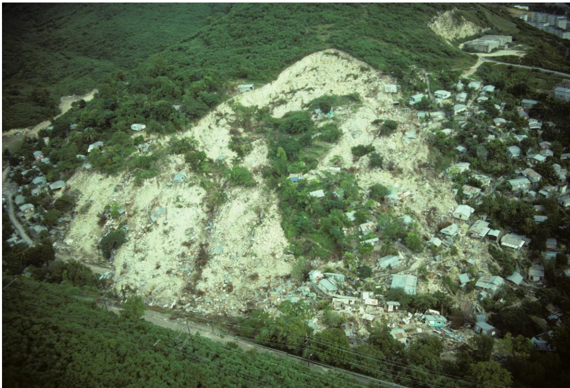
Figure 4. Unplanned community on steep unstable bedrock, Barrio Mameyes, Ponce, southern Puerto Rico. Photo source: R. Jibson, USGS, 1985. Hillslope failure killed 129 people (Jibson, 1989).
