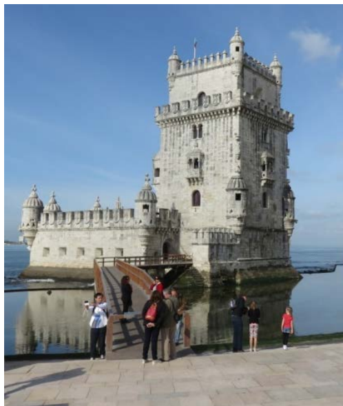
Figure 3. View of the east and north façade of the Tower de Belem in 2015. Note the regular soiling pattern that developed from water running down the holes in the round walk terrace. Photo Angelo Silveira, DGPC – DEPOF archive.
