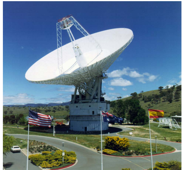
Fig. 9. The 70-m antenna of the Canberra Deep Space Communications Complex, located outside Canberra, Australia. This complex is one of three that comprise NASA's Deep Space Network. The other complexes are located in Goldstone, CA, and Madrid, Spain. (NASA photograph.)
