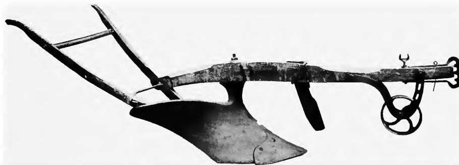
FIGURE 6.—Eagle plow, about 1849. (Catalog No. 54.)
