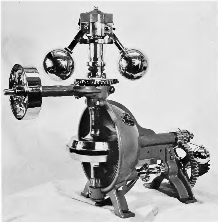
FIGURE 43a.—Woodward "Type 3" water turbine governor, 1903. (NMHT 315896. Smithsonian photo 45926-J.)
