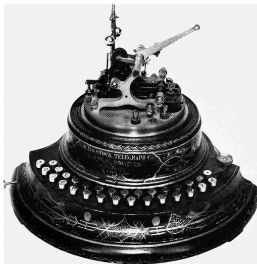
FIGURE 77.—Patent model of Thomas A. Edison's Gold and Stock printing telegraph, 1873. (NMHT 252616. Smithsonian photo 71882.)
