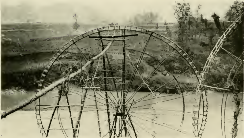
2. A large waterwheel made of bamboo and used for irrigation in Sze-huan. The wheel is propelled by the force of the stream.
