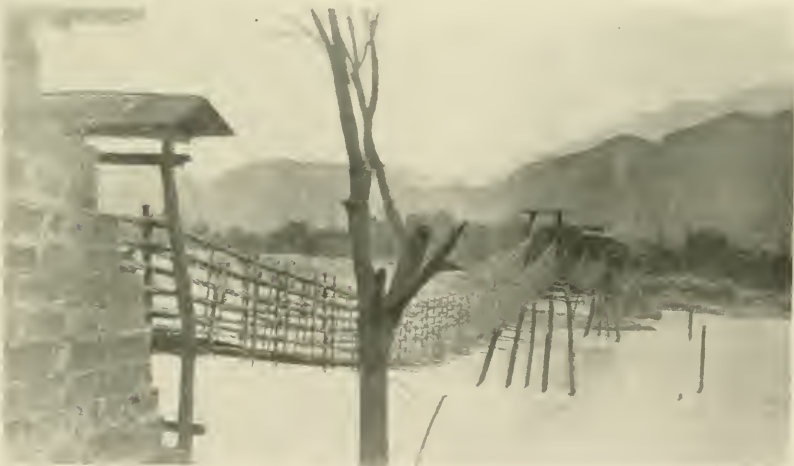
2. A great bridge made of large bamboo ropes or cables at Kuanshien, Szechuan, China.
