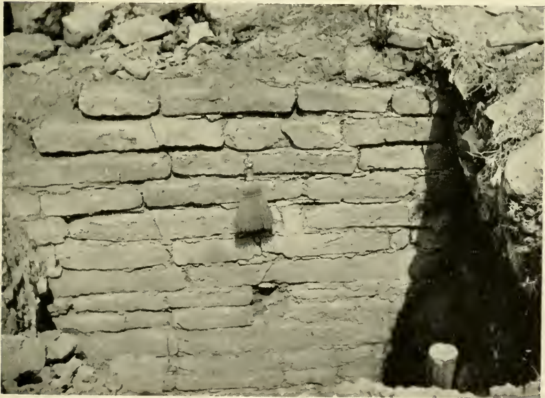
2. A typical section of Pinedale masonry. The second slab below the whisk broom is 4 feet long.
