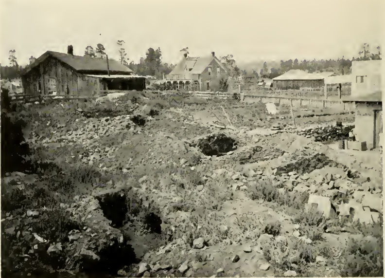
1. Showlow. The diggings at the right are tests 1, 2, 3, and 12 where the excavated rooms were found superimposed upon older structures.
