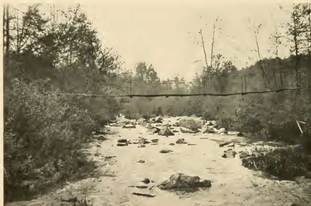
2. Hardware River, near the crossing of the old Lynchburg road, showing a primitive suspension footbridge high above the water.
